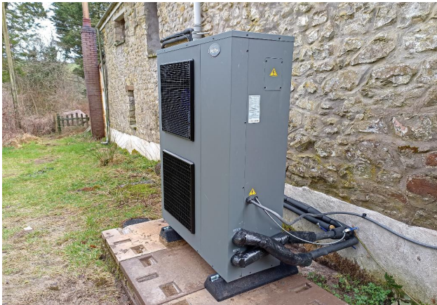
New Air Source Heat Pump
