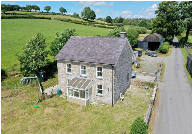
Main Aerial View 1
