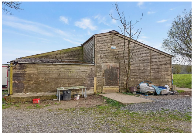
Front View Of Workshop
