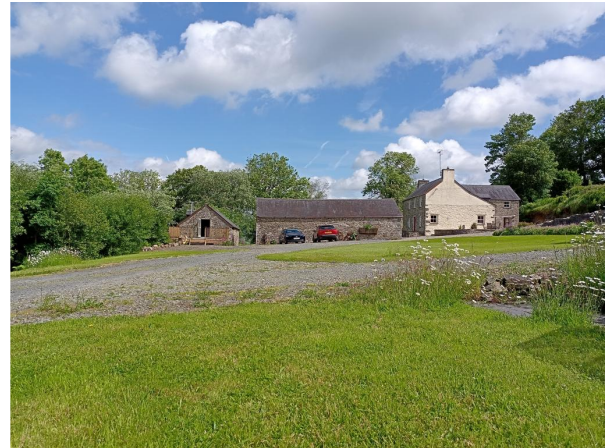
House And Outbuildings
