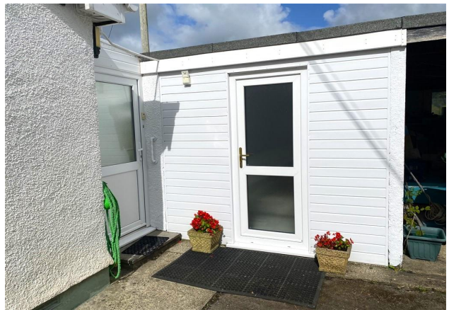
Entrance To Utility Building
