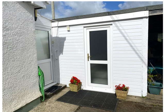
Entrance To Utility Building
