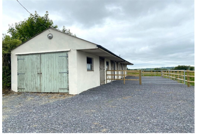
Stable Block And Hardstanding
