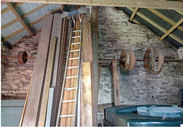
View Showing Old Mill Pulleys
