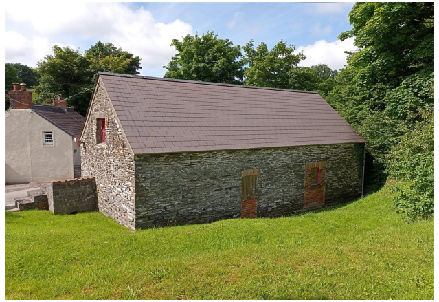
Rear View Of Barn
