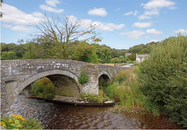
Bridge and Church In Nevern Village
