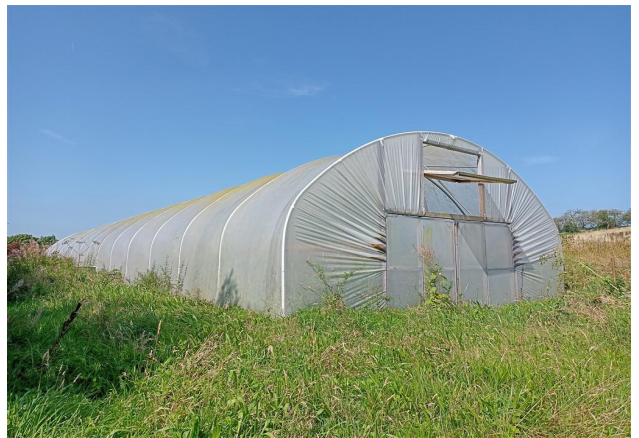
The Huge Polytunnel -View 2
