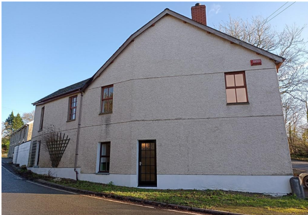
View Showing Workshop To Left Hand Side
