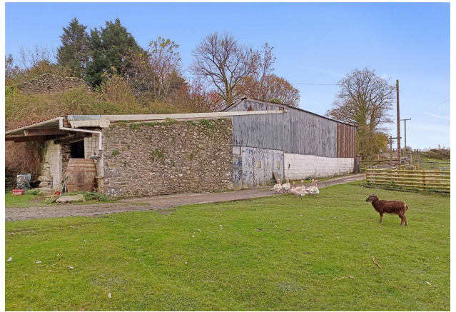
Main Outbuilding (subdivided)
