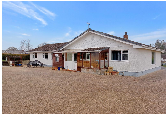
Rear View Of Bungalow
