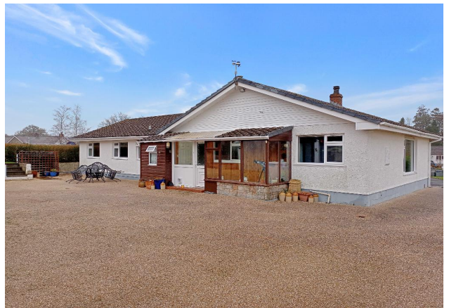
Rear View Of Bungalow
