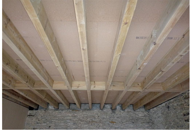
Bed 1 - New Joists And Flooring
