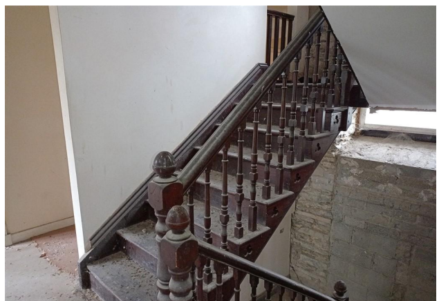
First Floor Landing
