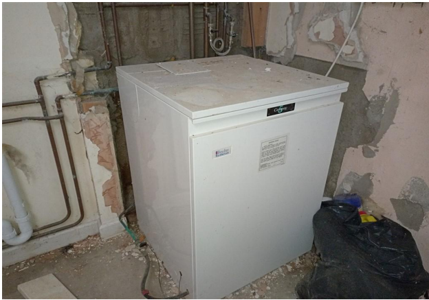
Floor Standing Oil Boiler
