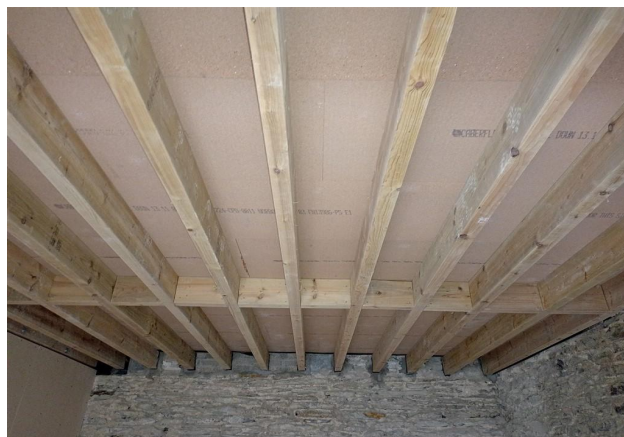
Bed 1 - New Joists And Flooring
