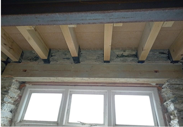
New Beam And Joists Fitted-Bed 1
