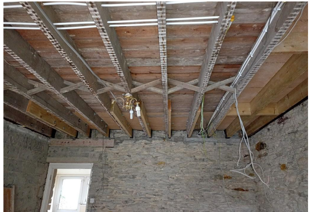
Lounge Ceiling-Some New Joists
