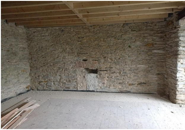
Bedroom 1 - New Ceiling/Joists
