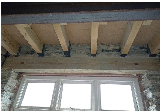
New Beam And Joists Fitted-Bed 1
