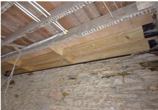
Lounge Ceiling - New Joists
