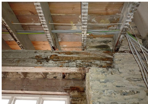
Two Rotten Structural Beams
